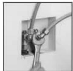
Fig. 19 - Terminal union between the hydraulic taking and the radiator
