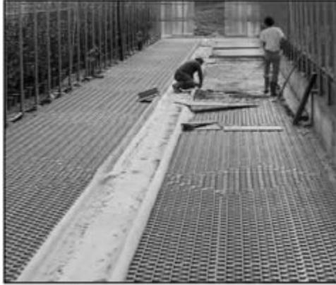
Fig. 22 - Installation of FILTERMO pipe for a heating floor system
