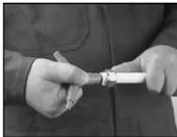
Fig 10. Pipe calibration
